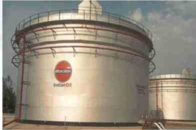
Cone / Dome Roof Tanks
