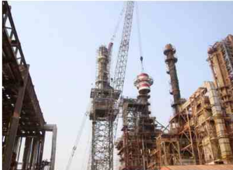
Maintenance, Shut Down / Revamp
