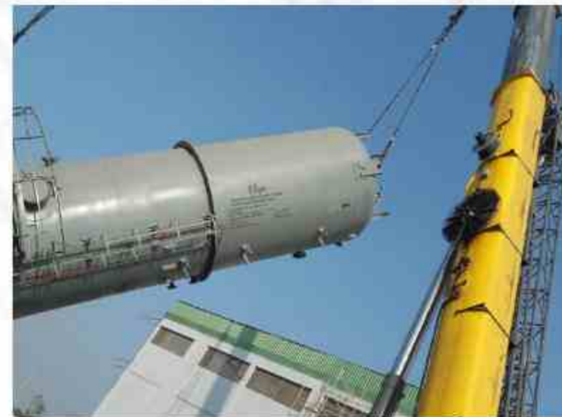
Fabrication & Erection of Equipments
